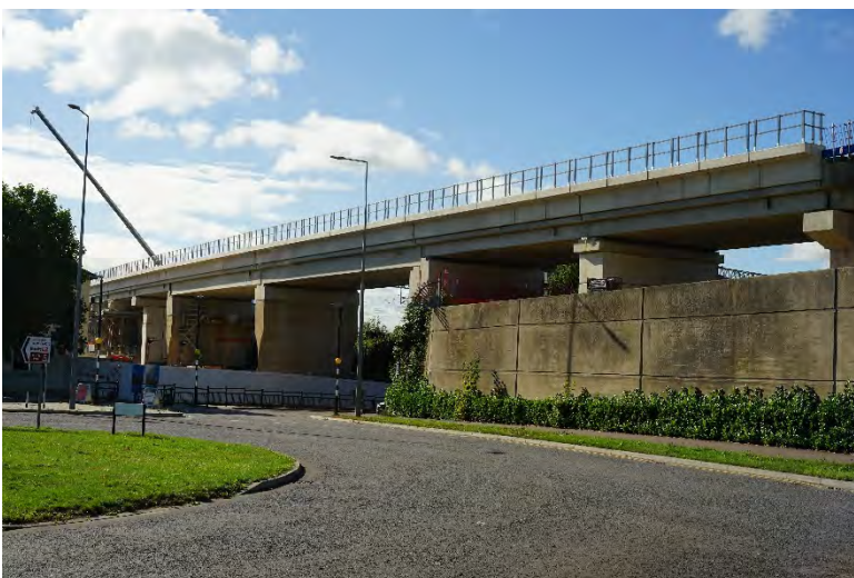
Bletchley Flyover over Buckingham Road
